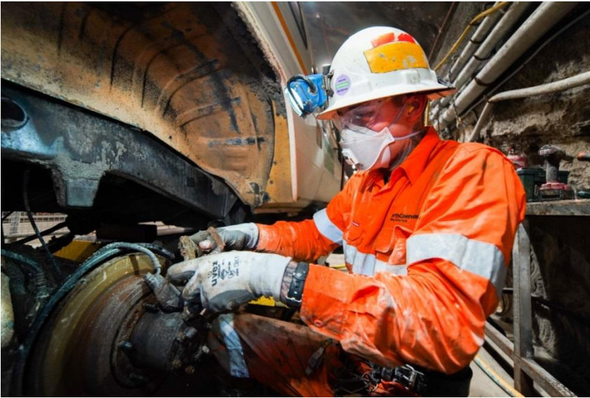
The first roadheader being demobilised
