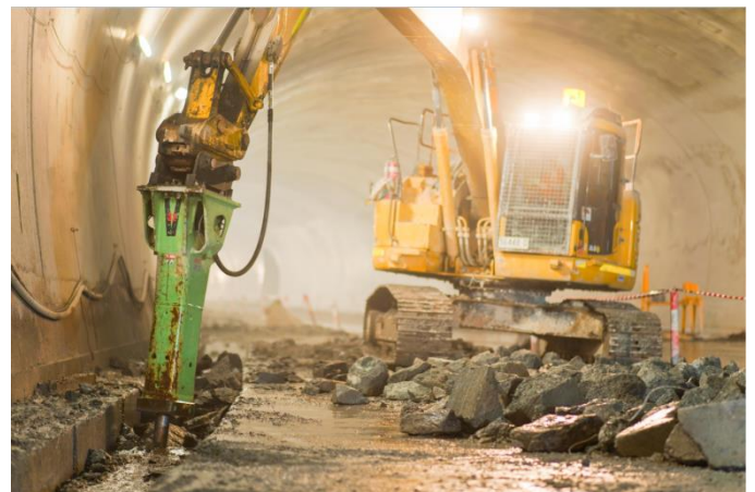
Trenching - excavation of troughs to house services
