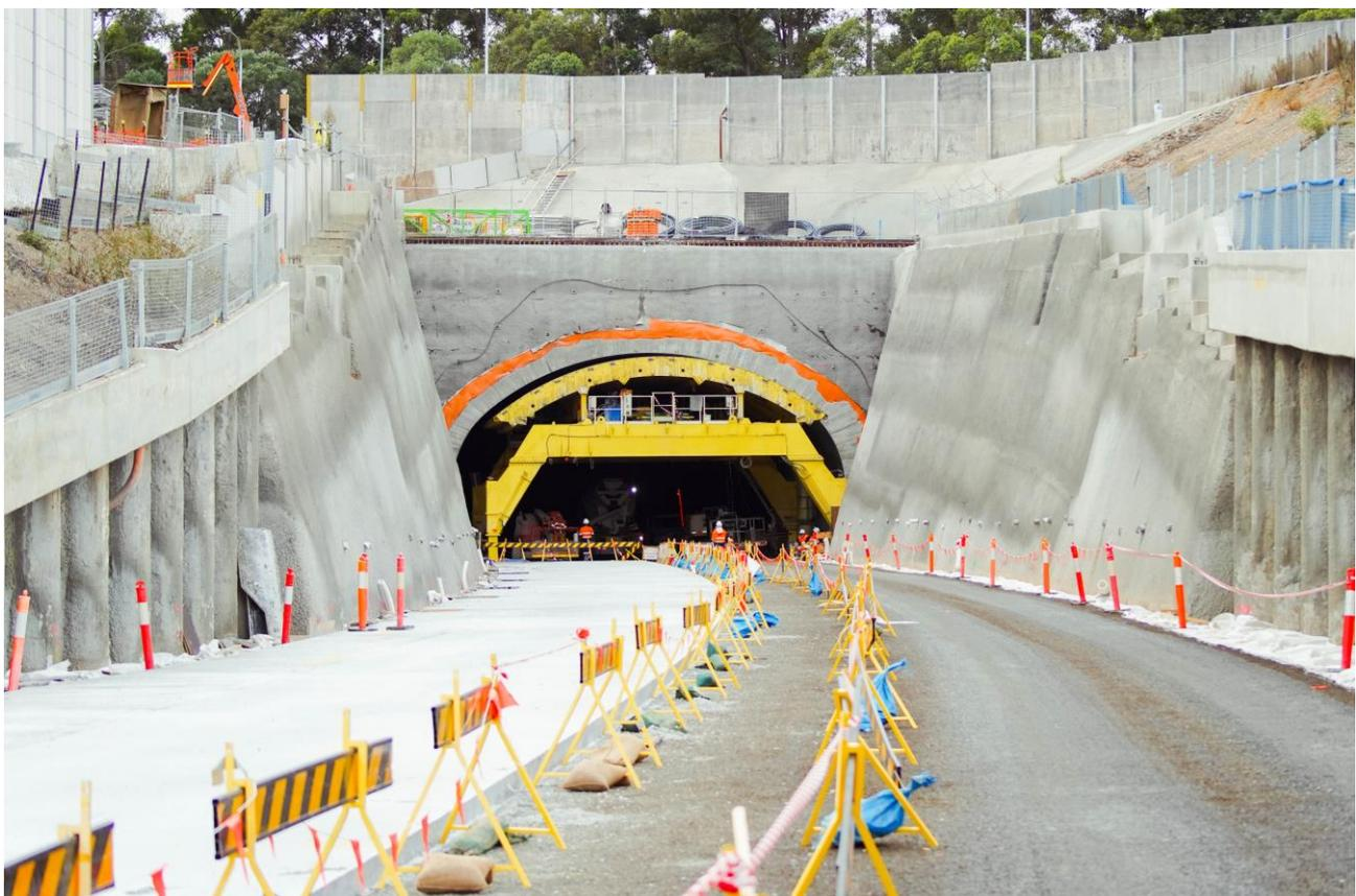
A gantry is used to install the final lining for the northbound tunnel entry accessed from the Hills M2 Motorway.
